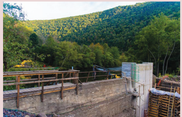
Progress is beautiful at the Mansion House Bridge construction when captured by Board Member, Mike Burnside.
