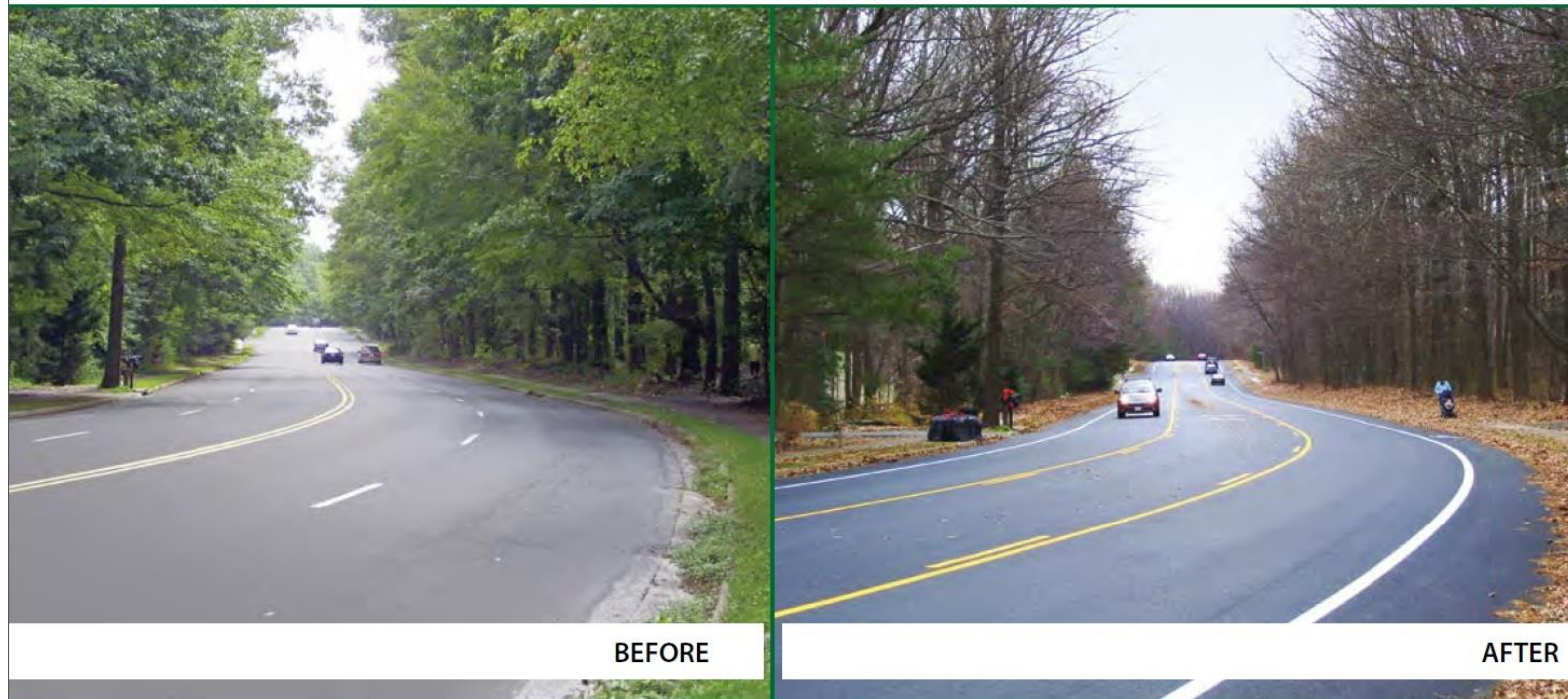
Figure 1. Road Diet Photo Credit: Virginia Department of Transportation
