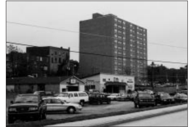
Rear elevations are often neglected and tend to be avoided.
