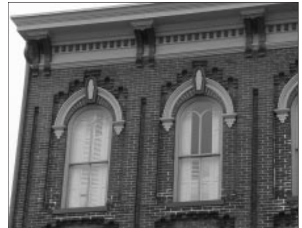
Many upper floors along Main Street retain original architectural elements.
