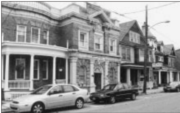
Lansford retains a majority of its historic architecture.
