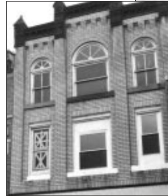
Original windows have been shortened on the second floor. Third floor windows retain original fanlights (left). Inappropriate window replacement alter the appearance on the left side of this building (right).
