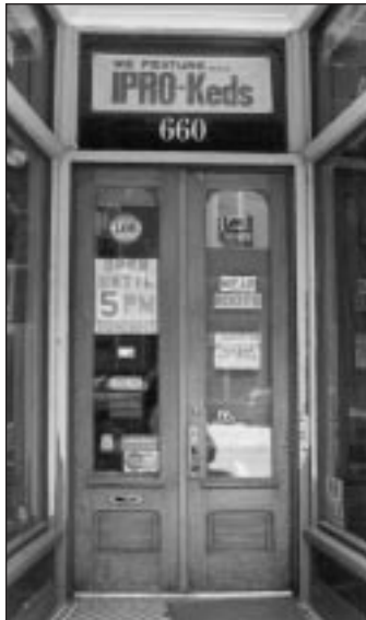
Original double-leaf doors should be retained.
