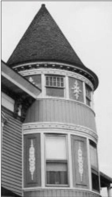
A variety of roof shapes are found in the region.
