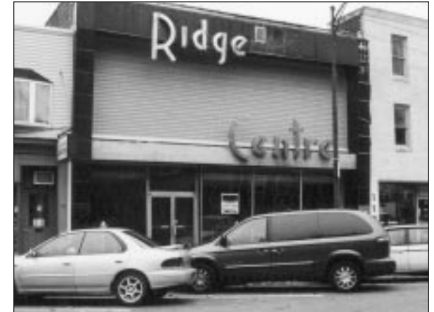
Structural glass panels are found on the Ridge Centre Building, Lansford.
