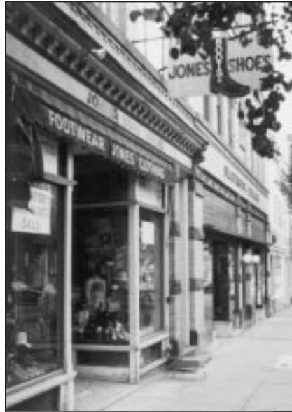
This storefront retains its 19th and early 20th century features including display windows, recessed doorway, bulkhead, cornice, piers, signage, awning and terrazzo tiled entry.
