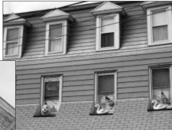
This mansard roof has been insensitively covered with siding (above). Maintaining architectural elements is critical. Covering or removing damaged architectural detail such as the cornice at left should be avoided.
