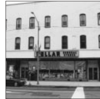
Architectural cornices have been removed from some Lehigh buildings.
