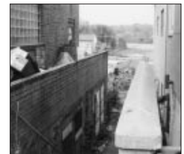
Alleyways connecting First Street to rear parking areas should be improved.
