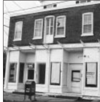
Although windows have been shortened, this White Haven landmark retains most of its original storefront features.
