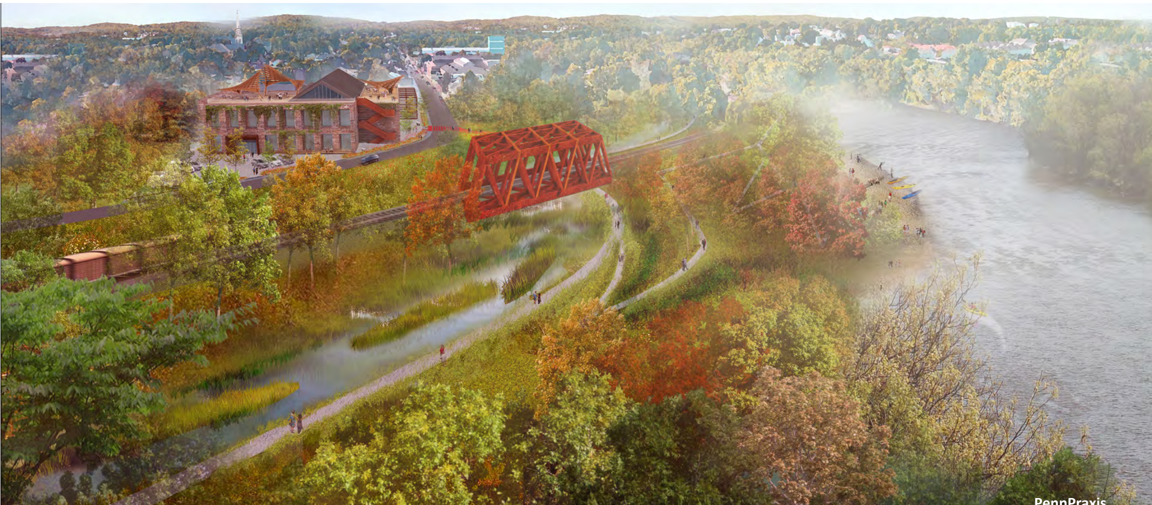
D&L TRAIL, WATER TREATMENT CANAL AND SILK MILL IN NORTH CATASAUQUA
