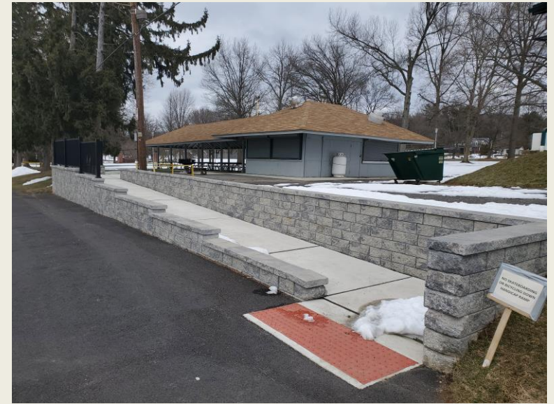
CDBG-funded ADA Access Ramp constructed at an old community park to provide access from the parking lot, over a swale, to the interior park paths
