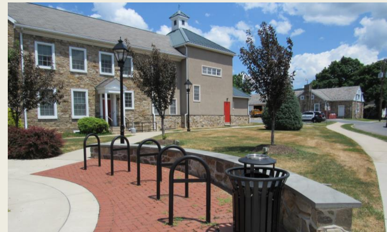
DCED-Funded Town Center Streetscape and Bicycle/Pedestrian Safety Improvements
